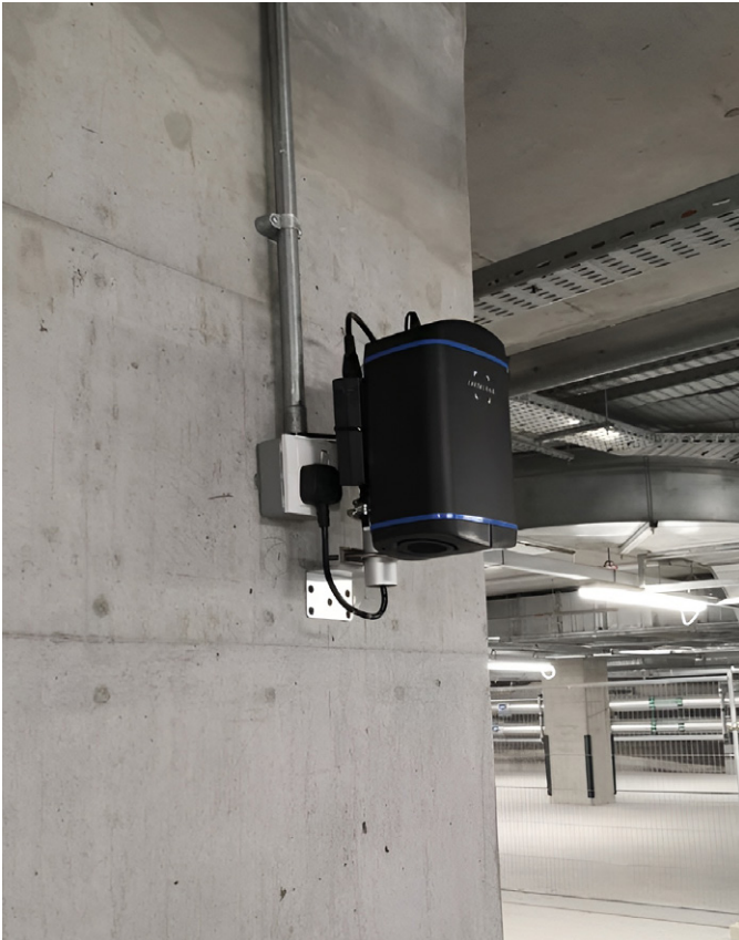
Figure 3: Mains powered Zephyr® deployed on a concrete wall in one of the underground areas at Expo 2020 Dubai.
